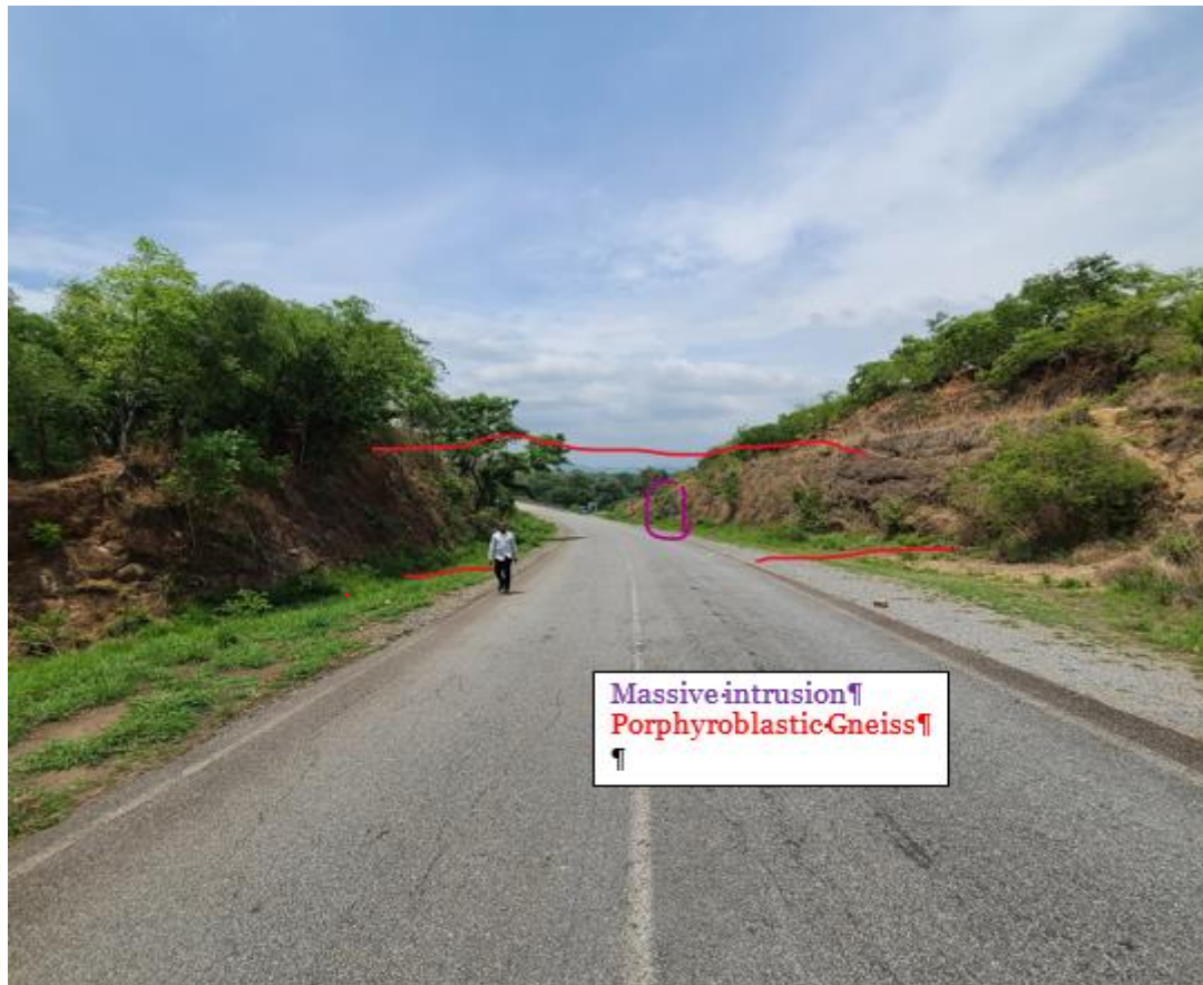
Figure 24. M005 road cutting through rock units at Mphalanyongo fault near Bua river.
