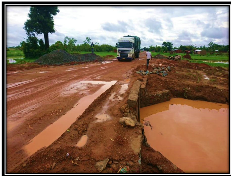
Figure 10. Reconstruction of washed away section near Mkaika Filling station: a deep gully formed a stream and washed away the section.
