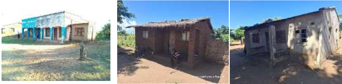
Figure 4-1: Examples of structures affected by the project
