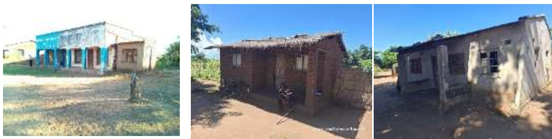
Figure 4-1: Examples of structures affected by the project
